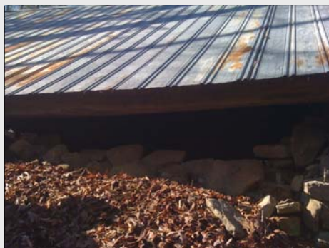
Façade of Pinckney's Tomb (above) and the east wall where stones have fallen due to pressure from tree roots.
