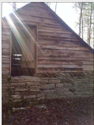
Façade of Pinckney's Tomb (above) and the east wall where stones have fallen due to pressure from tree roots.
